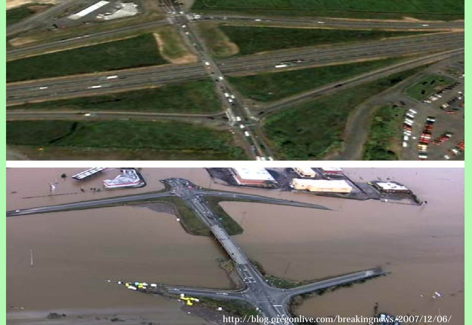
Figure D: Google image showing Interstate 5 at Chehalis before the flood paired with stills from video shot on December 4, 2007.
